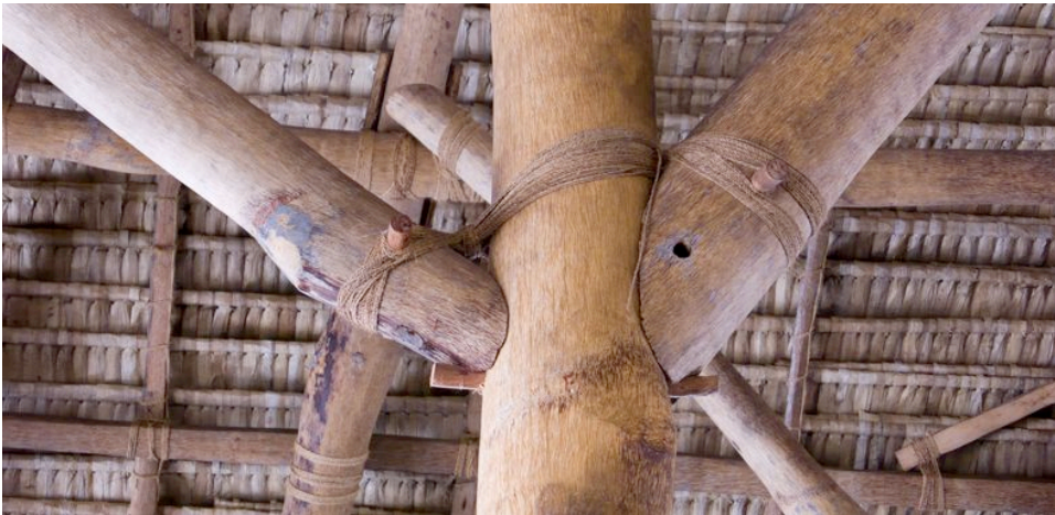
Figure 11 – No nails or screws are used in construction, only lashings and wooden pegs
