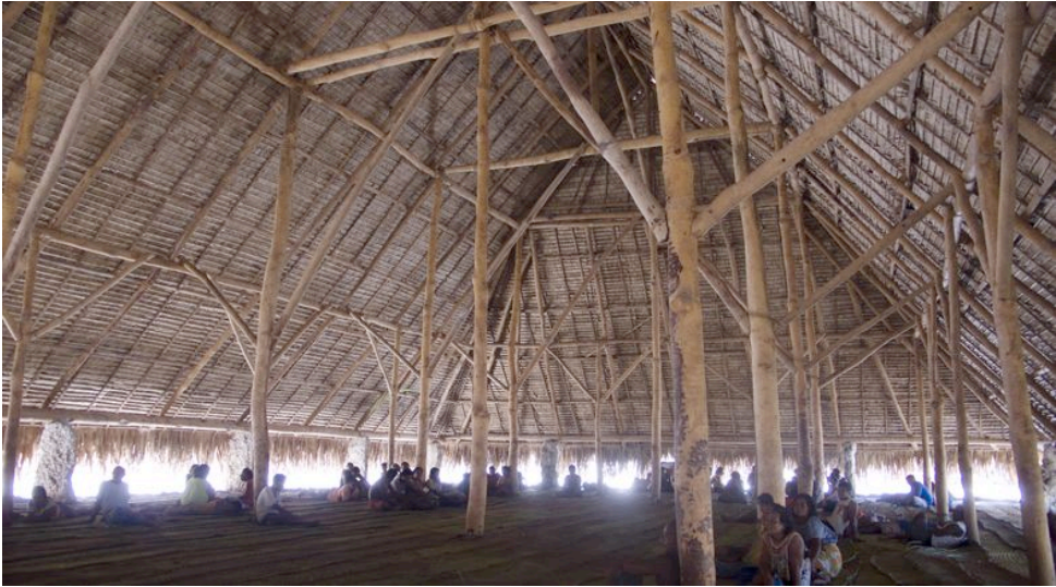
Figure 10 - Burenneita Mwaneaba at Eita village on Tabiteuea North
