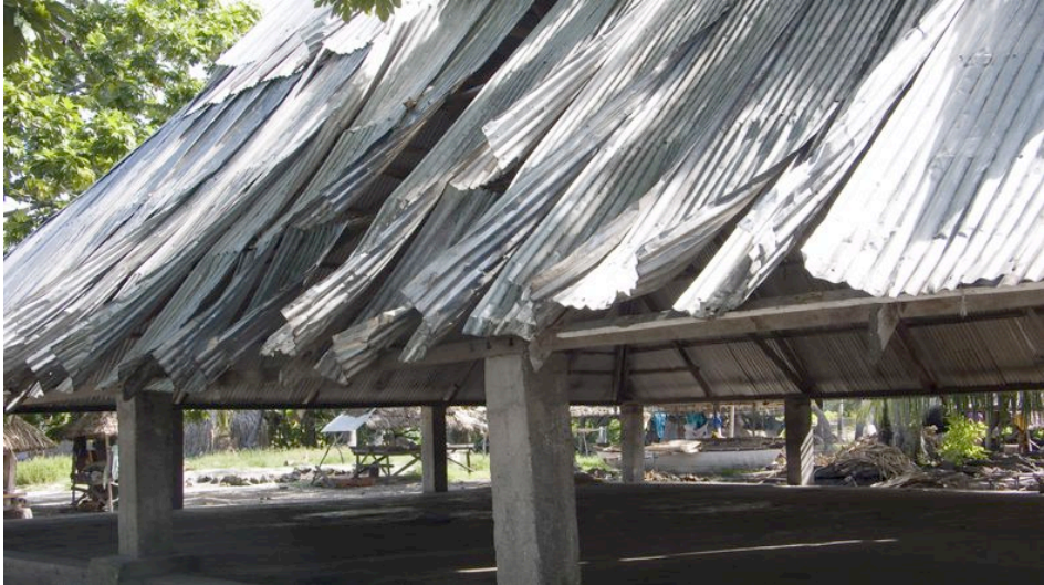
Figure 19 - An iron roof torn by strong winds awaits 'aid' funding for replacement
