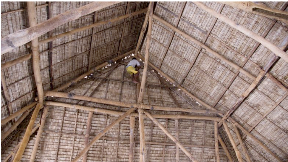
Figure 9 – Working with skill and courage in the roof of te mwaneaba
