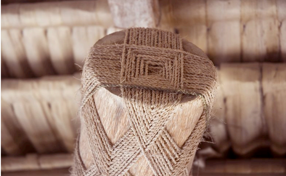
Figure 6 – Sophisticated knots and lashings made from local string are joint-specific
