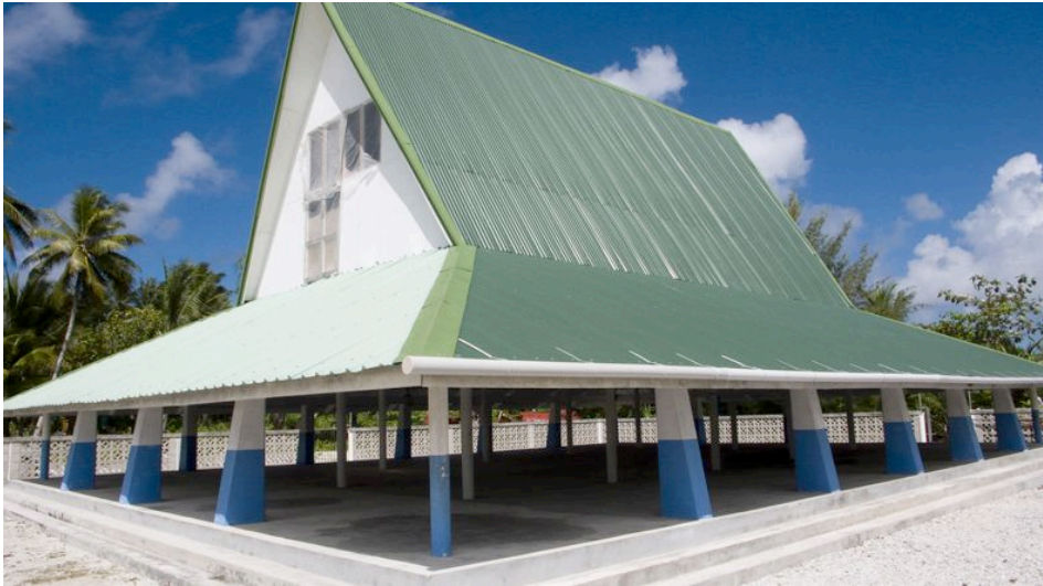
Figures 13, 14 and 15 - South Tarawa mwaneaba constructed of imported materials
